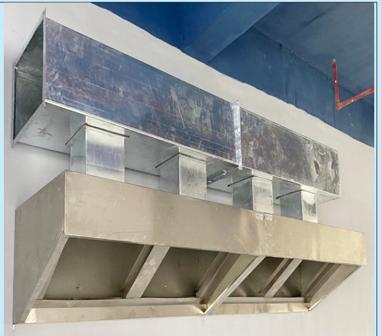
SS CHIMNEY WORKS
